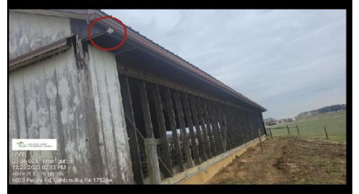
Why? Gutters that are not connected to downspout provide no stormwater control as runoff is intended to be routed to an appropriate outlet.
