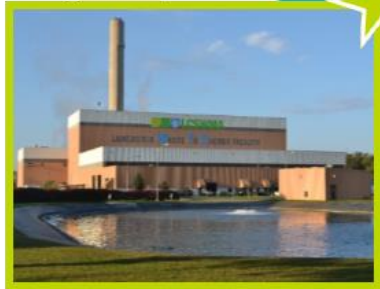
Lancaster WTE Facility 1,200 TPD
