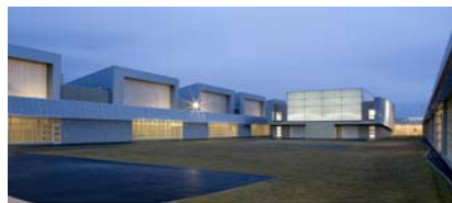
Union County Juvenile Detention Center. Credit: JINGOLI
